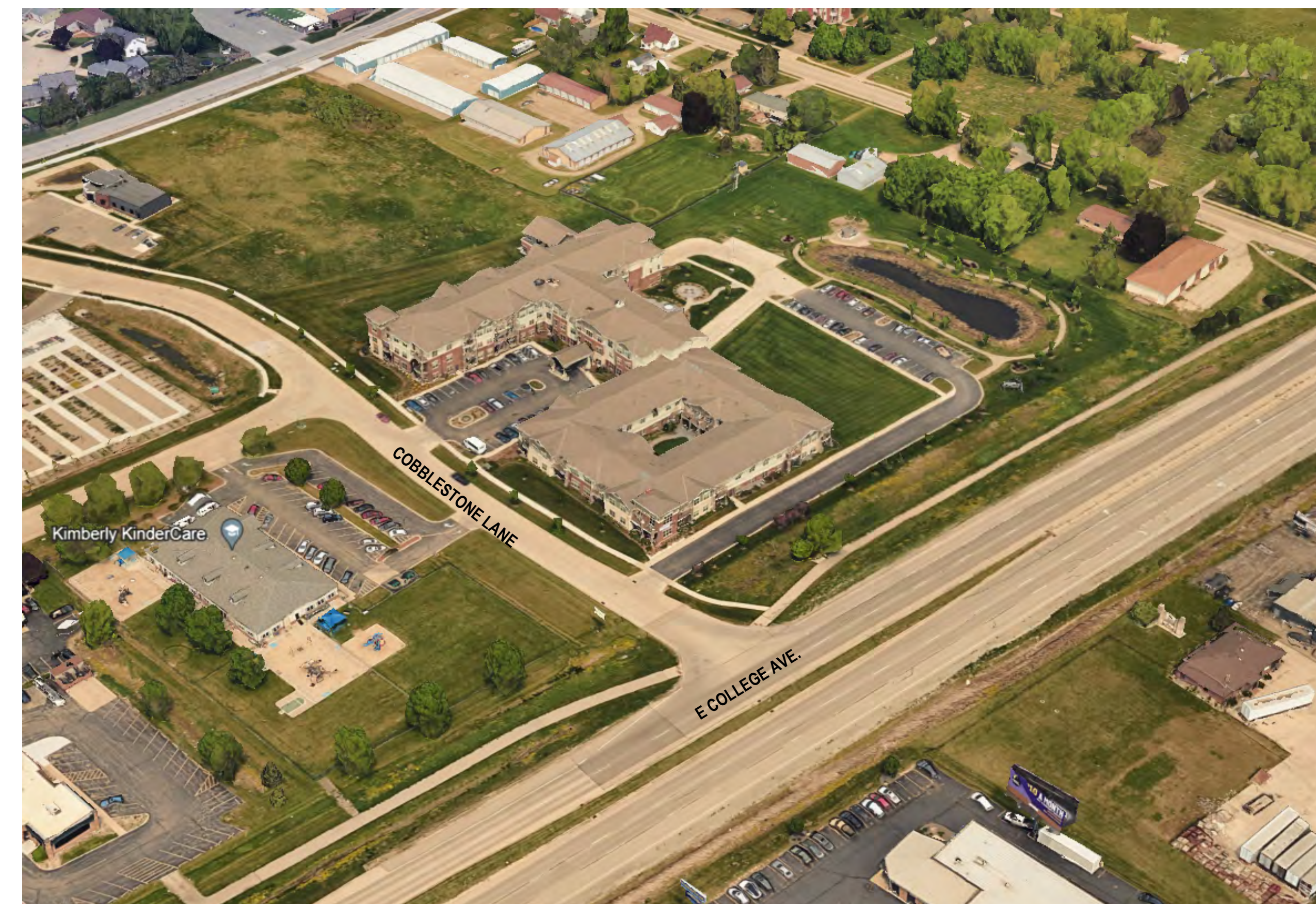
7. Aerial view of existing site
