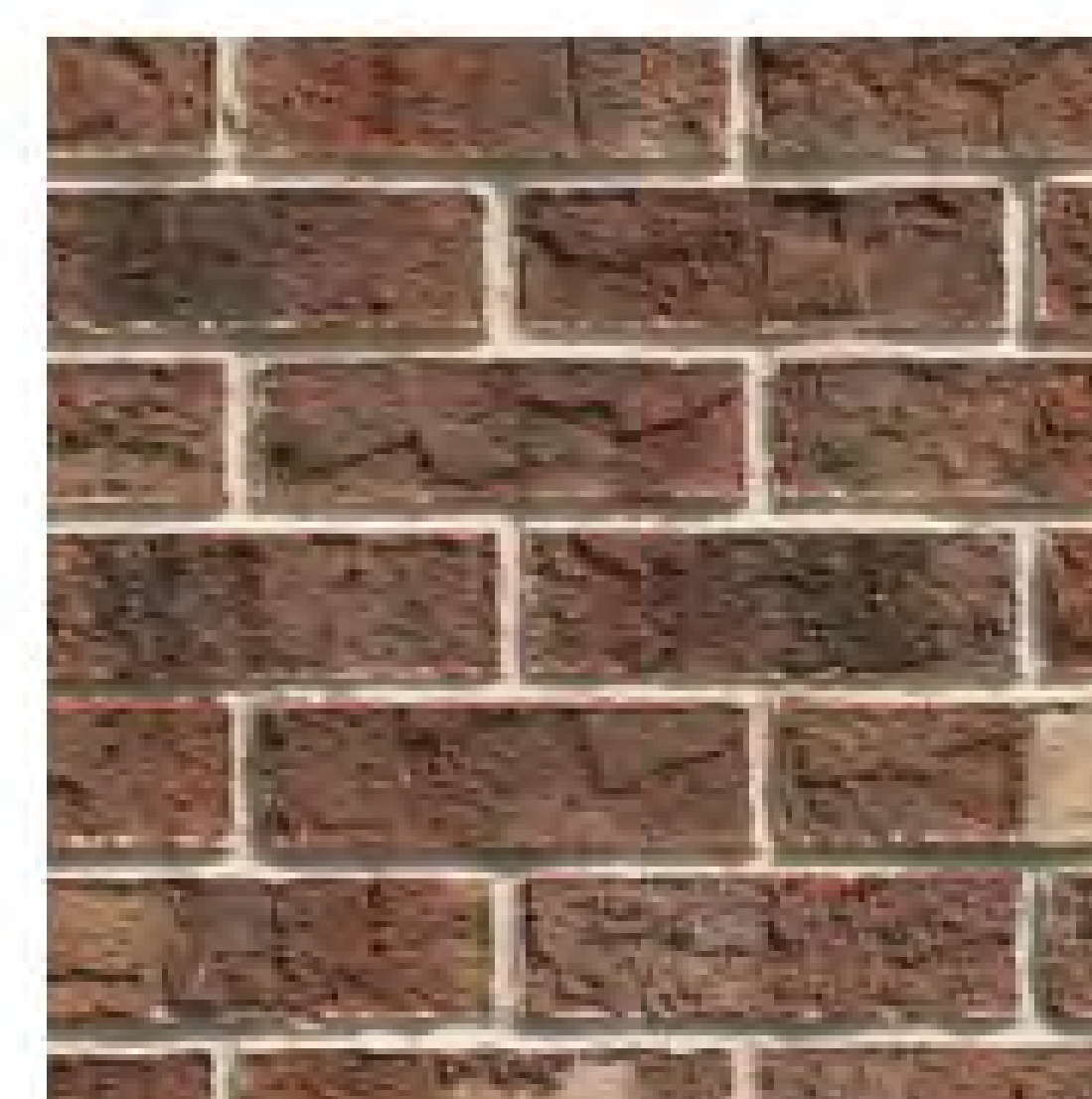
COUNTY MATERIALS TRIANGLE BRICK NORTHHAMPTON UTILITY
