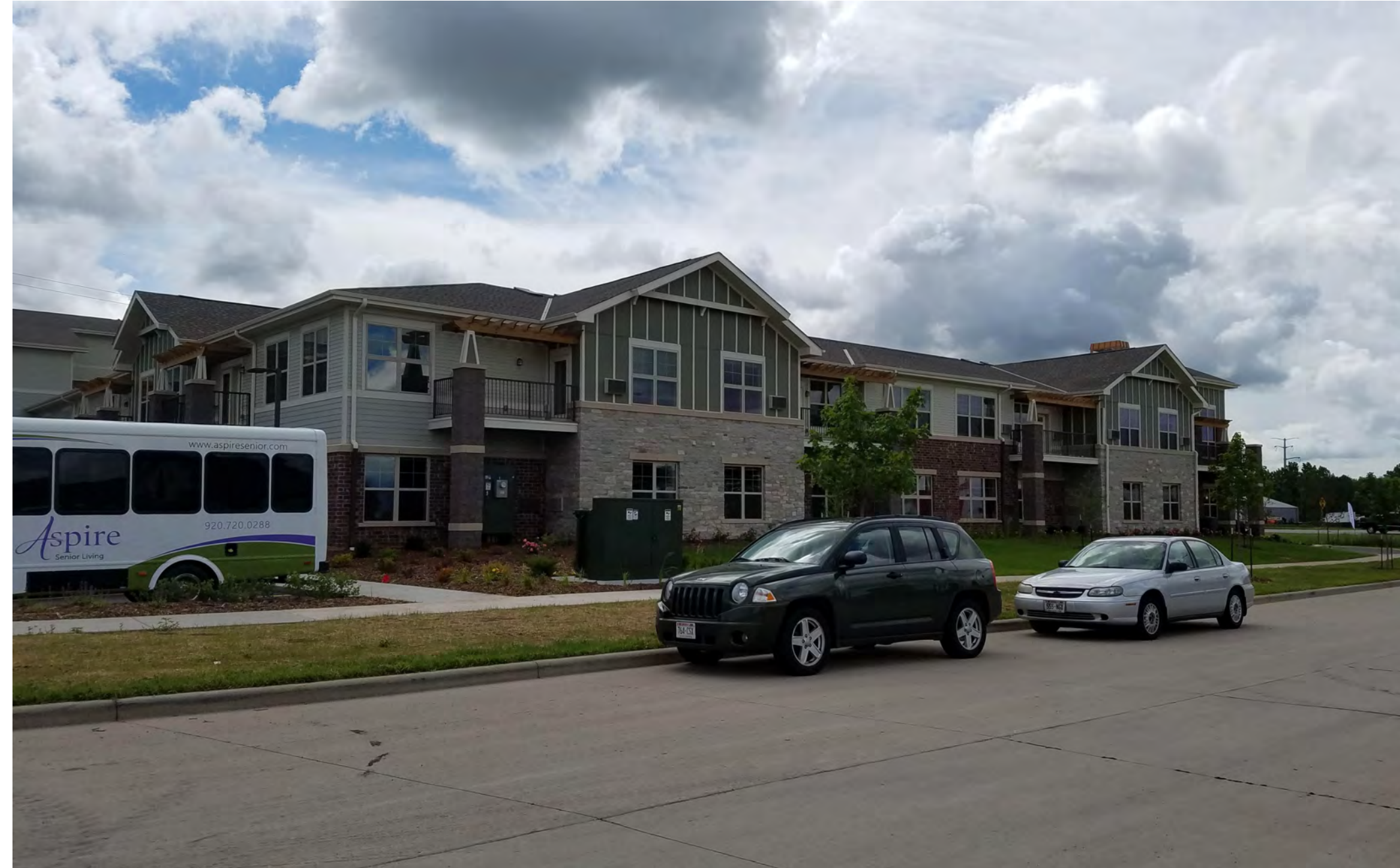
2. Northwest corner of assisted living wing seen from Truman St.
