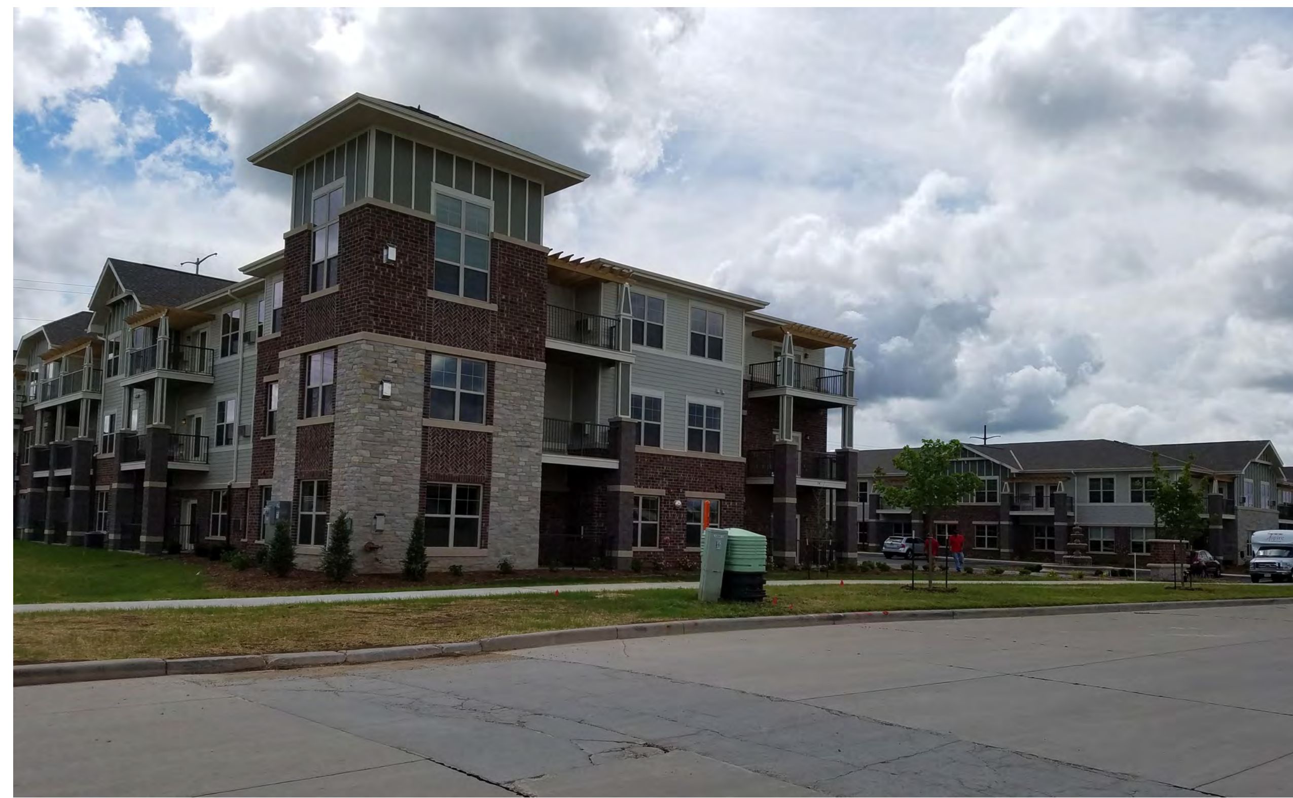
5. Northwest corner of independent living wing seen from Truman St.
