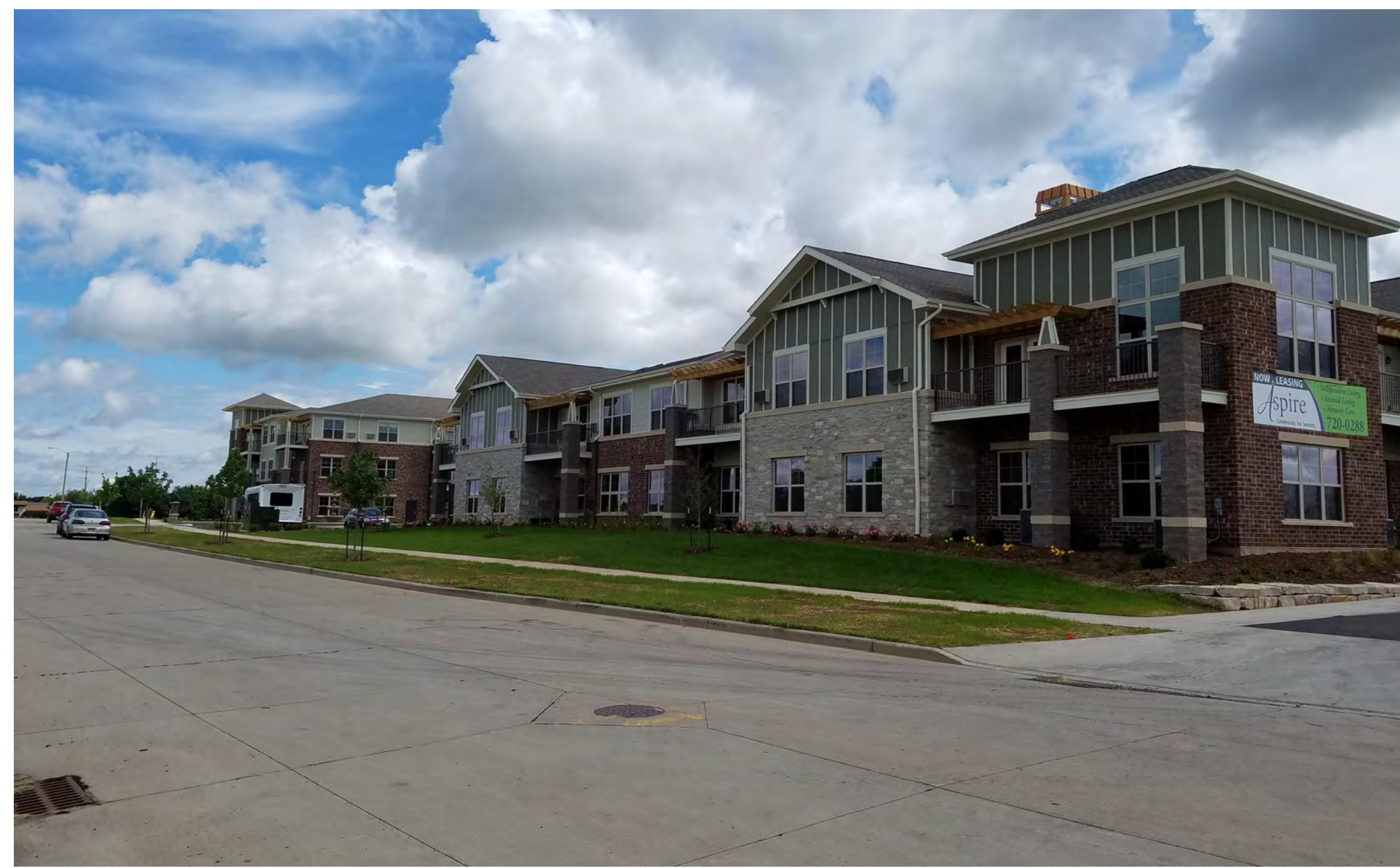
1. Southwest corner of assisted living wing seen from Truman St.
